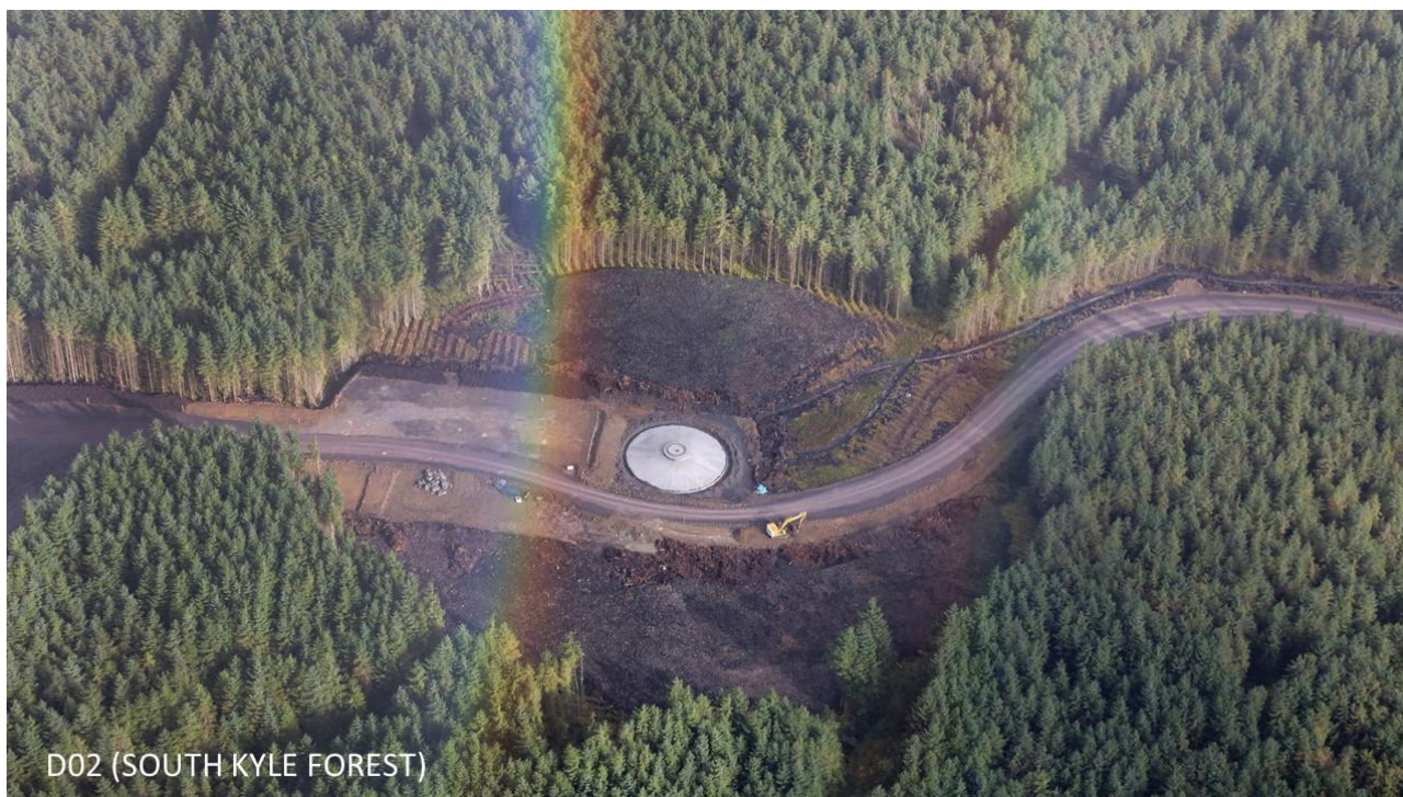
Diagram 3.1: Concrete turbine foundation (South Kyle Wind Farm)
