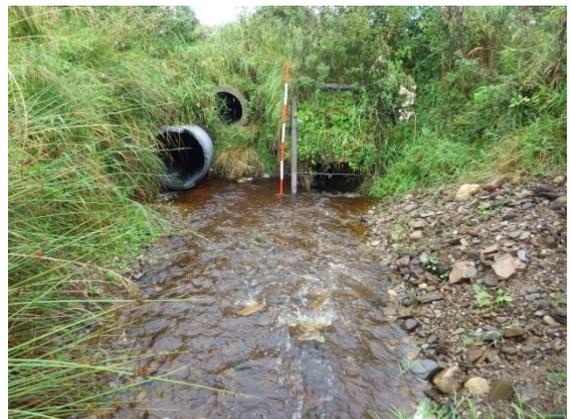
**Plate 12 – AM6 (triple culvert / impassable)**
