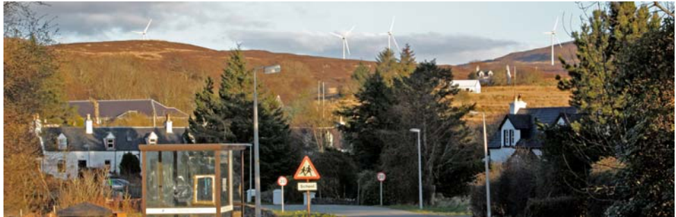
The wind farm viewed from Edinbane village
