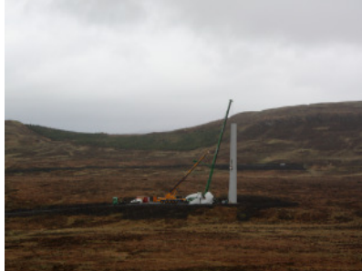
The tower sections are raised into vertical position
