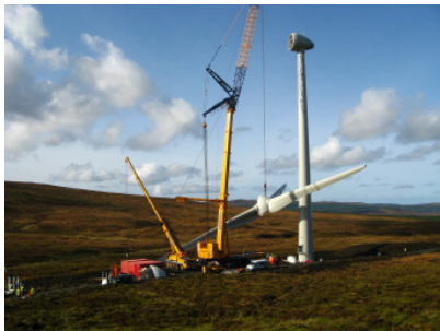
The rotor assembly is lifted into position
